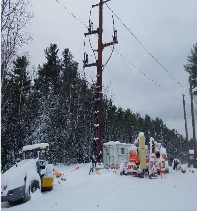
Fig 1: Str. 99 at Getchell property/west side of the Bay. Viewing west. (12-02-19).
