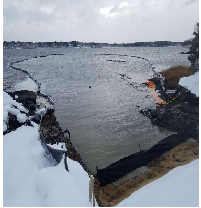
Fig 2: Turbidity curtain at Getchell property/west side of the Bay. Viewing east. (12-02-19).
