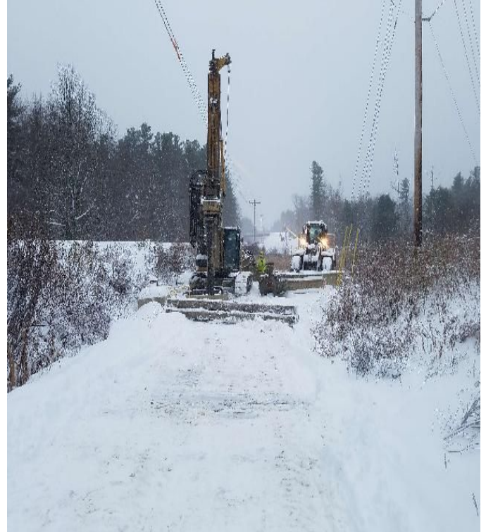
Fig 4: Drilling foundation for Str. 2. Viewing south. (12-03-19).
