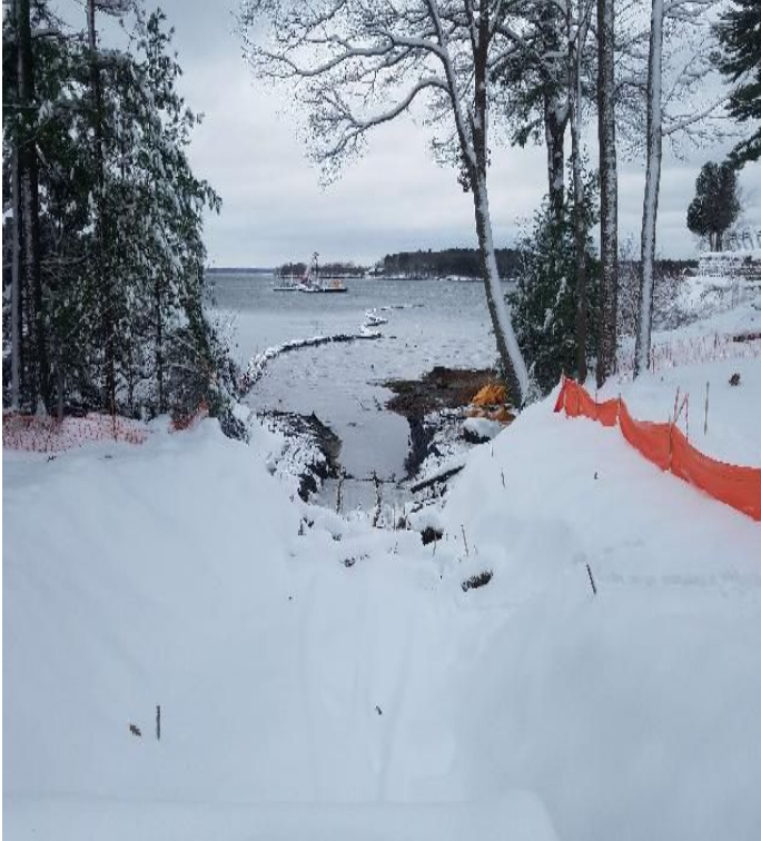
Fig 3: Trench and turbidity curtain at Gundalow landing/east side of the Bay. Viewing southwest. (12-02-19).
